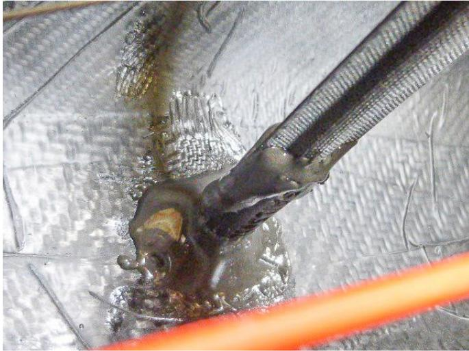
When the filler has partly cured, coat your fingers with liquid soap and smooth the roughly formed filler to make a smoother surface. If the resin is too soft to do this come back to it after another 30 minutes. Access to the lower end of the tube may be difficult in the confined space of the bow.
