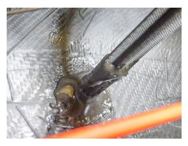
When the filler has partly cured, coat your fingers with liquid soap and smooth the roughly formed filler to make a smoother surface. If the resin is too soft to do this come back to it after another 30 minutes. Access to the lower end of the tube may be difficult in the confined space of the bow.
